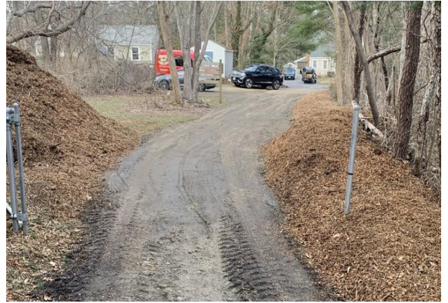
Mulch spread along the sides of road to ball court to create a berm and help prevent washout.
