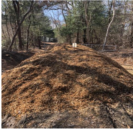
Mulch spread along the sides of road to ball court to create a berm and help prevent washout.
