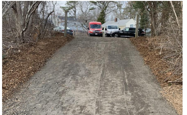
Slope to ball field widened and graded for safety and to help prevent washout.
